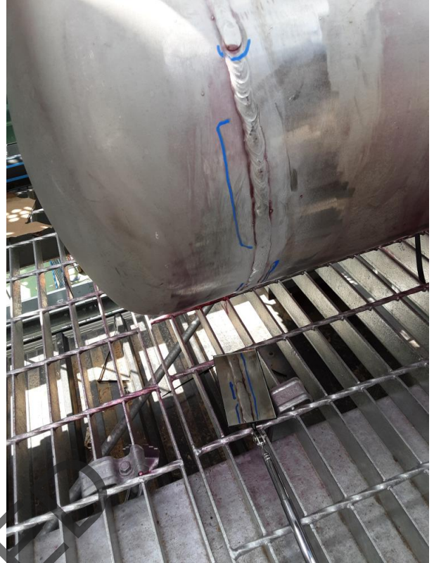
Image 2 of 13 - BTM SP3 W1: Lack of fusion areas 7-10 o'clock facing north
