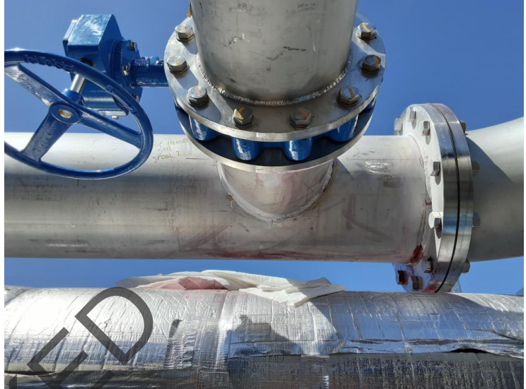
Image 6 of 9 - Top header South end spool #2 W7-9
