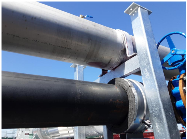
Image 8 of 9 - Top header South end spool #3 W6
