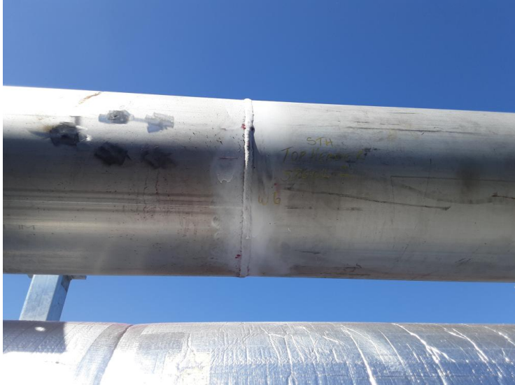
Image 5 of 9 - Top header South end spool #2 W6
