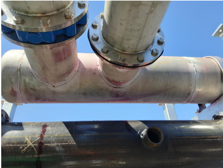
Image 1 of 9 - Top header South end spool #1 W1-6
