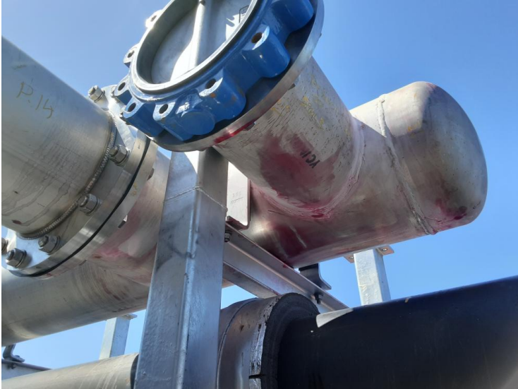
Image 9 of 9 - Top header South end spool #3 W7-11
