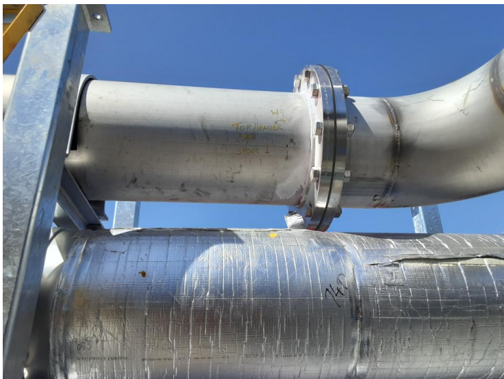
Image 3 of 9 - Top header South end spool #1 W9
