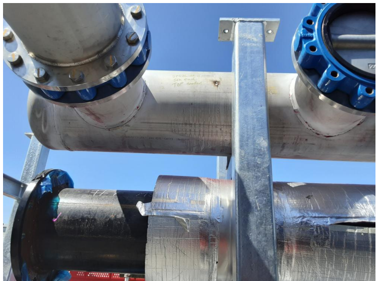
Image 4 of 9 - Top header South end spool #2 W1-5
