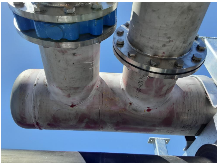
Image 7 of 9 - Top header South end spool #3 W1-5
